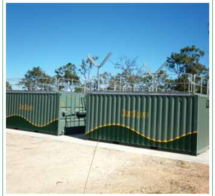
The Ozzi Kleen transportable containerised system is becoming the preferred treatment plant for mining and construction projects in remote locations – when delivered, the system can be installed and ready to operate quickly. The Ozzi Kleen transportable containerised range is available in many configurations with the modules in parallel or in series to cater for higher BOD and hydraulic loadings.
